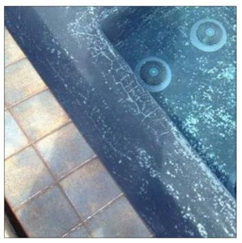
streaks, blotchy) deterioration and discoloration of cement flatwork applications, such as pool plaster.
